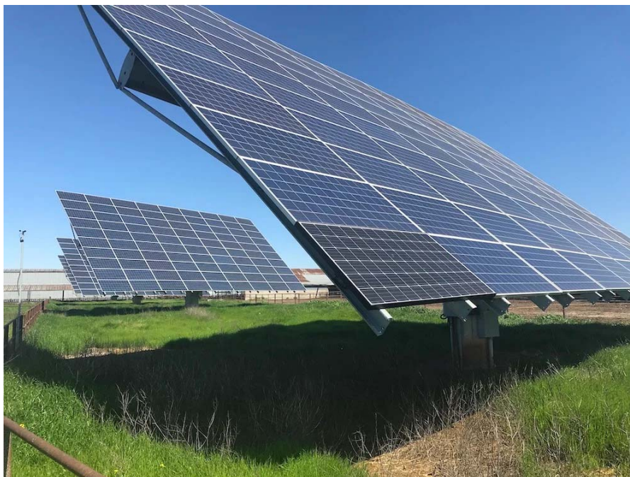
Large format dual axis trackers capture more late afternoon light. Credit Charles W. Thurston
